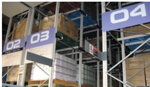
Automated warehouse at the Tsurugashima Site
