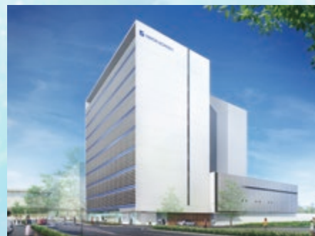
Image of the completed R&D facility
