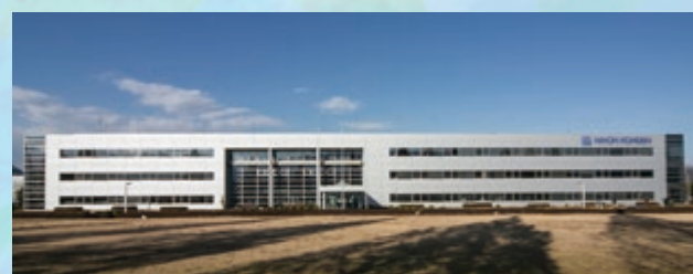
Image of the completed Tomioka Production Center
