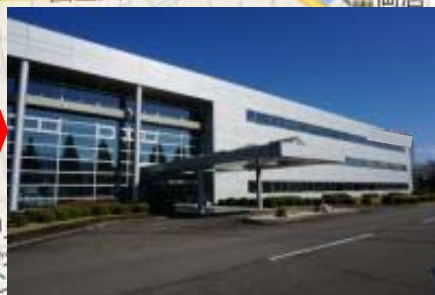
New plant Approx. 26,000m 2
