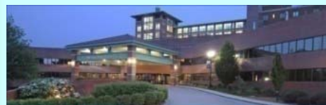
Holy Name Medical Center installed Prefense in early 2011
