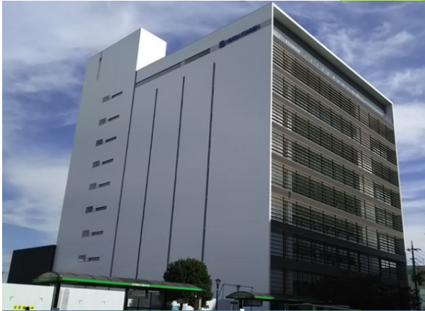
Advanced Technology Center
